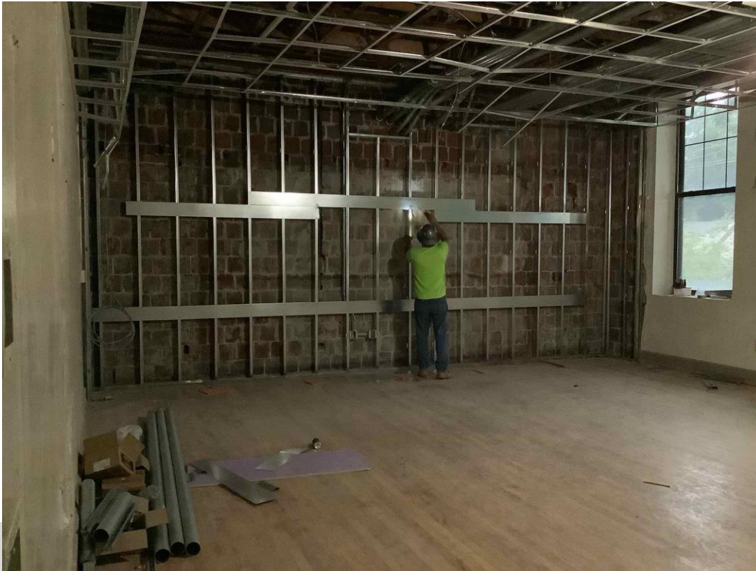
Interior framing at area B
