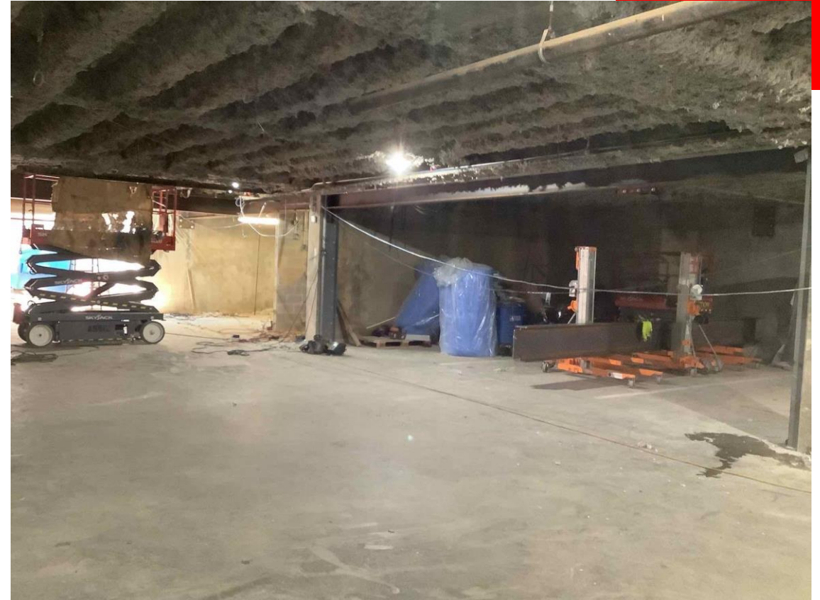
Structural steel installation at parking garage
